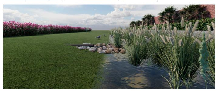
The underdrained bioswales along the road are the perfect answer to resolve the water logging issues, which often create those nasty traffic jams soon after a light rain. Here, rainwater has to filter through the plantation beds or gets discharged through pipe connection via French Drains.
